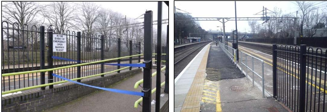
**Figure 5.6-3: Example of some temporary fencing that is obstructing access to the fast line platform (left). Examples of two types of fencing that were provided for reasons other than fatality prevention (right).**
