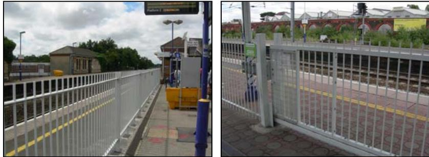
**Figure 5.6-1: Mid-platform fencing that has been installed at one of our trial stations (left). A sliding gate in the fencing to allow access to the platform when necessary (right).**
