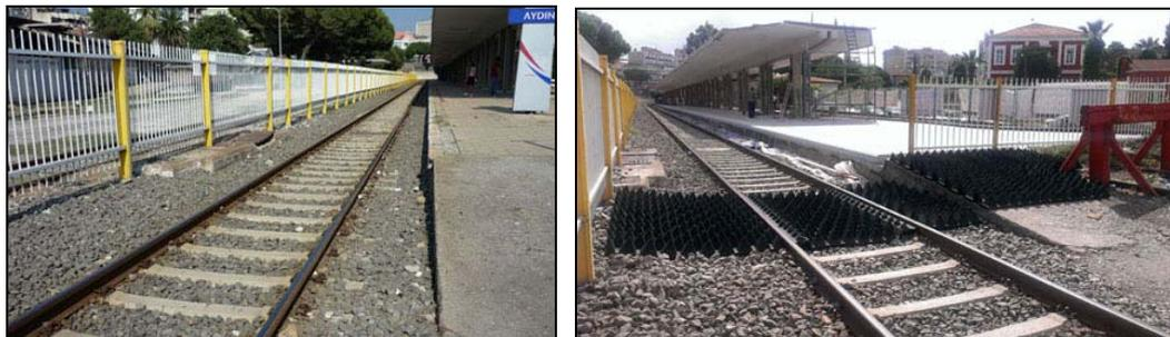
**Figure 5.5-7 Measure 7: Before/after Anti-trespass panels.**
