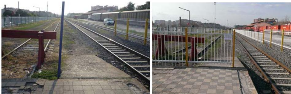
**Figure 5.5-8: Measures 2 and 3: Before/after Fencing.**
